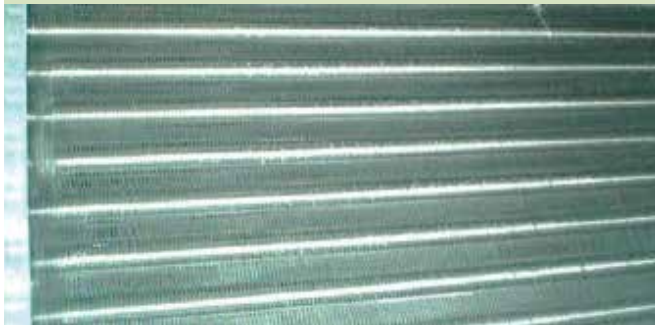
Clean Coil After HVAC Tune-Up
