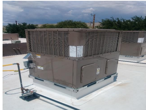
(Figure 1.2 Example picture of HVAC unit)
