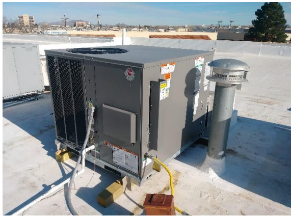
(Figure 1.1 Example picture of HVAC unit)
