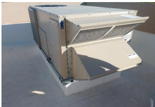
Figure 1.1 (Example picture of HVAC unit)
