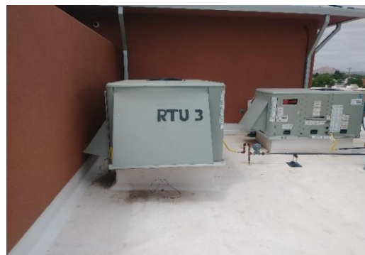
Figure 1.2 (Example picture of HVAC unit)
