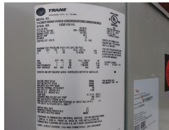
(Figure 1.8 Example picture of name plate of HVAC unit)
