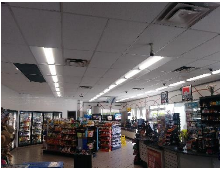
Figure 1.13 (Sample picture of ceiling fixtures)
