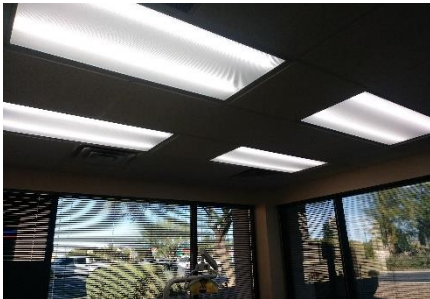
Figure 1.1 (Sample picture of ceiling fixtures)
