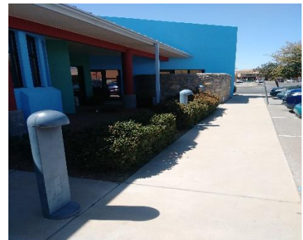
Figure 1.9 (Sample picture of exterior fixtures)
