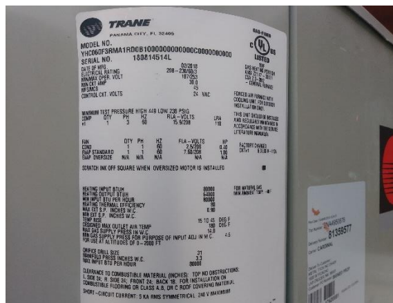
(Figure 1.8 Sample picture of HVAC unit nameplate)
