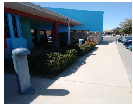
Figure 1.9 (Sample picture of exterior fixtures)
